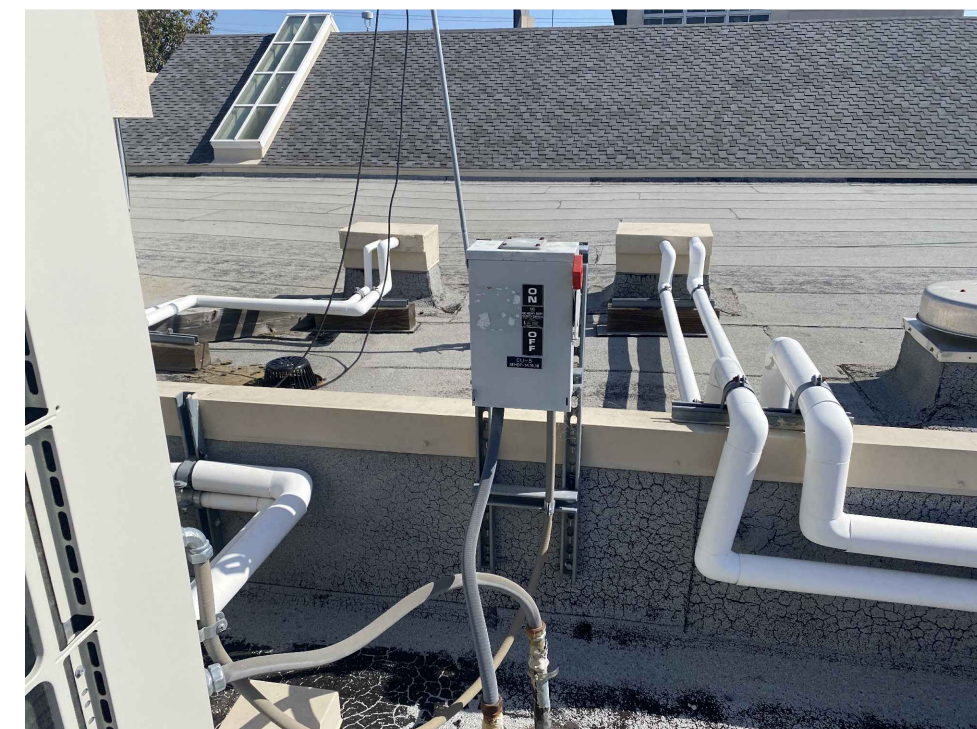
14 Pipe supports over parapet Refer 4/A2.3 and 8/2.3
