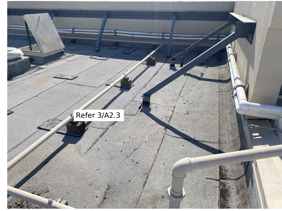
16 Accs. Hatch and parapet support Southwest corner
