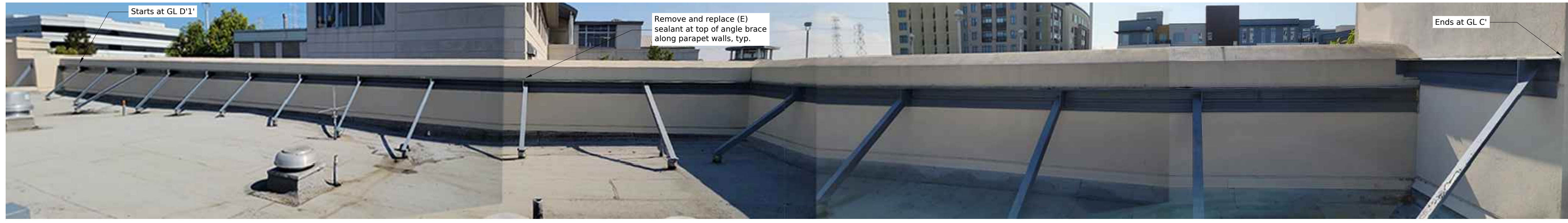
1 Angle Brace at parapet support
