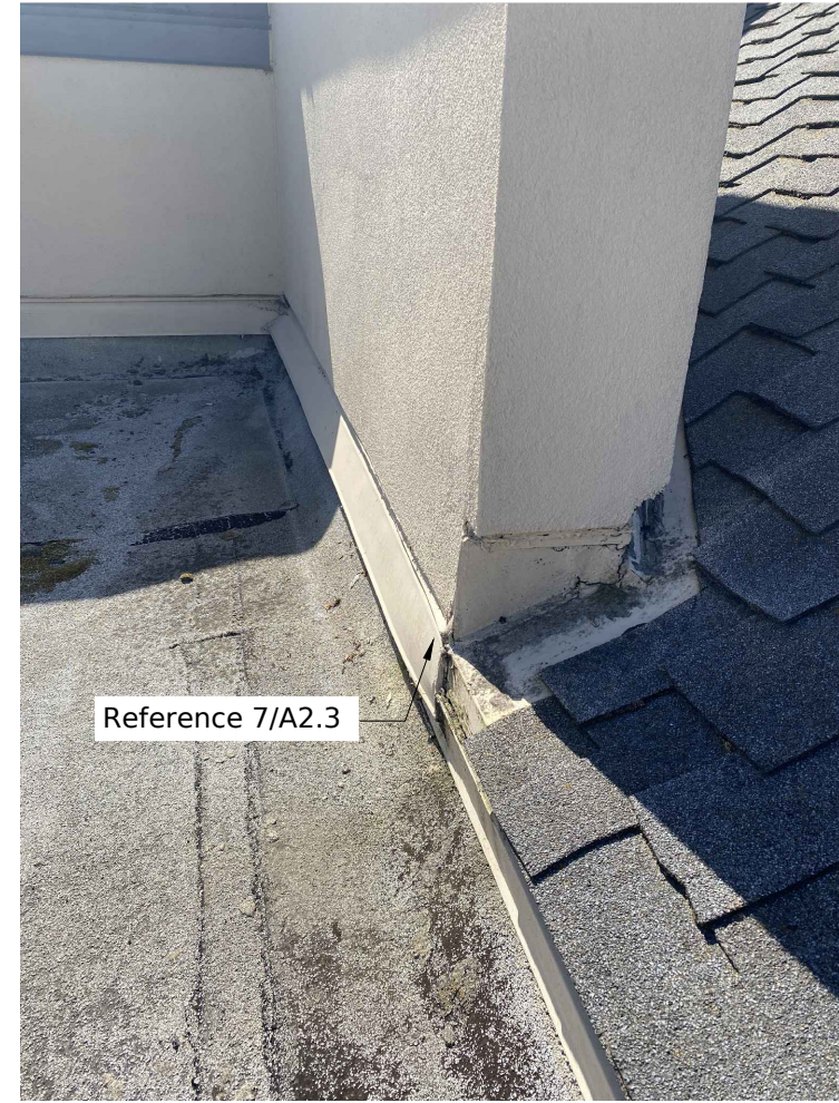
19 2 piece metal counterflashing typ.
