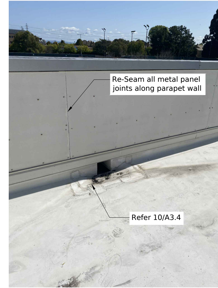
Through-Wall Scupper Along GL C, typ.
