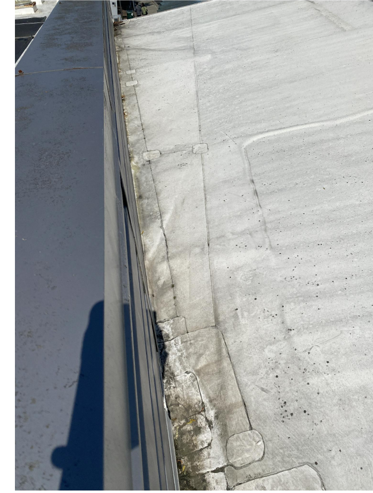
Lower Roof At GL B between GL 3 & 4
