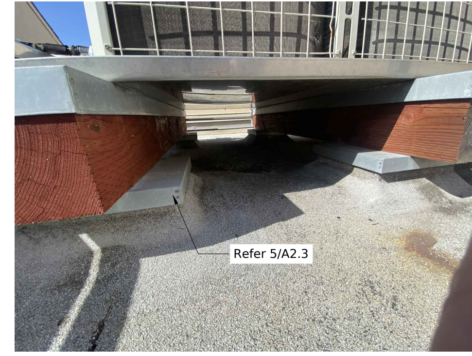
8 Mechanical curb typ.
