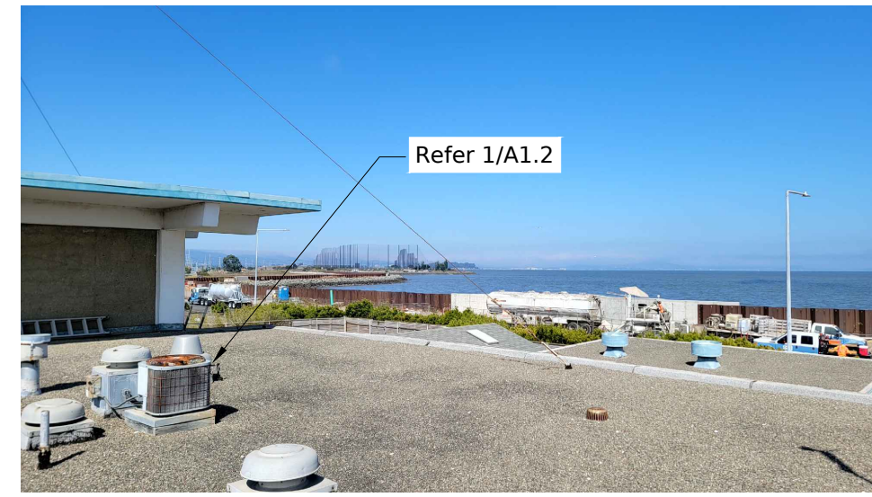
Pump Station Building
