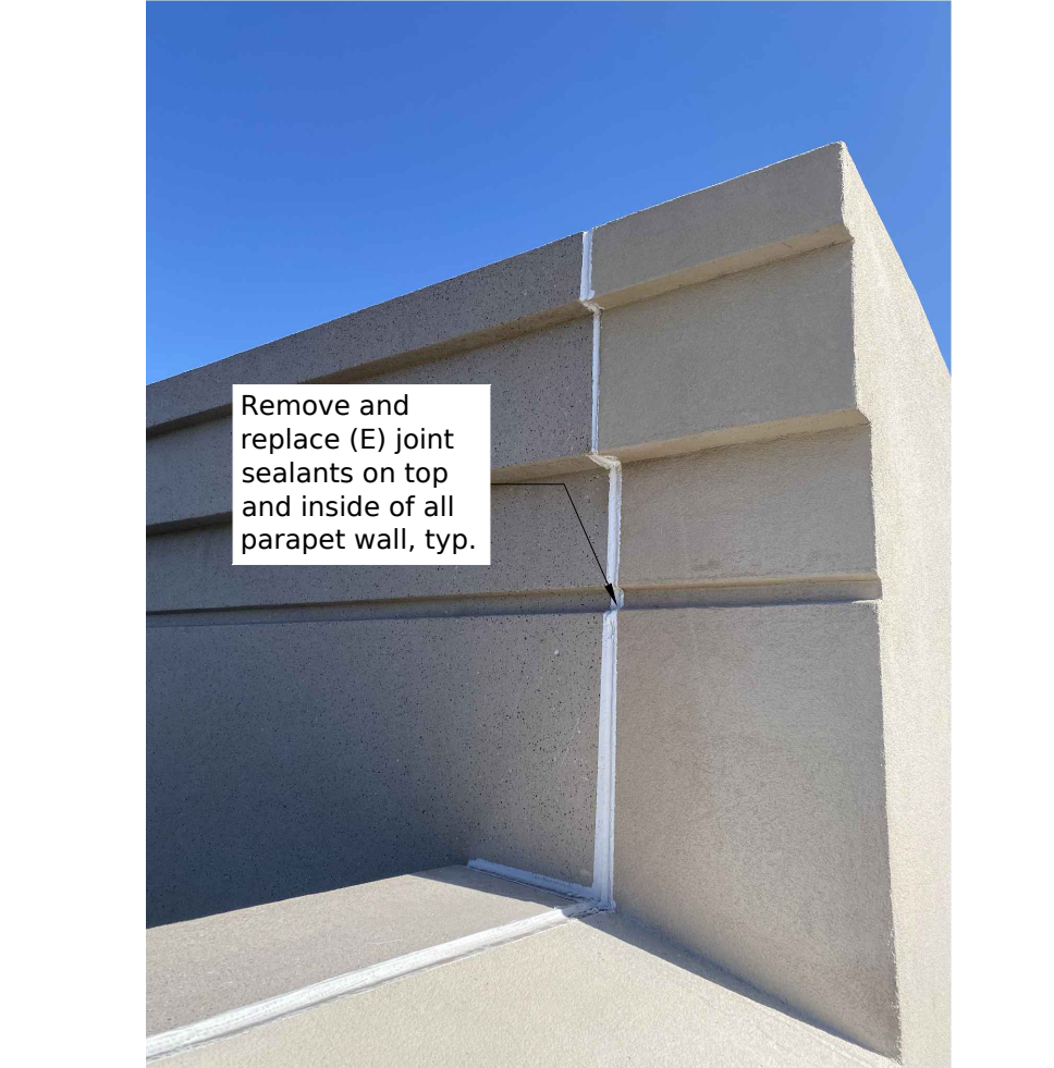
10 Parapet joint North and West edge of bldg.
