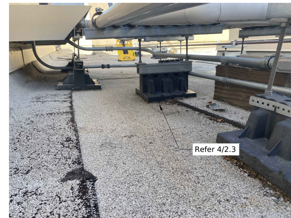
6 Pipe supports North area between GL B' and C' NTS
