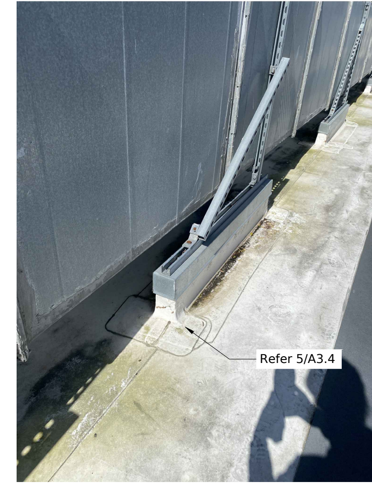
7 Lightweight Equipment Support Curb typ.
