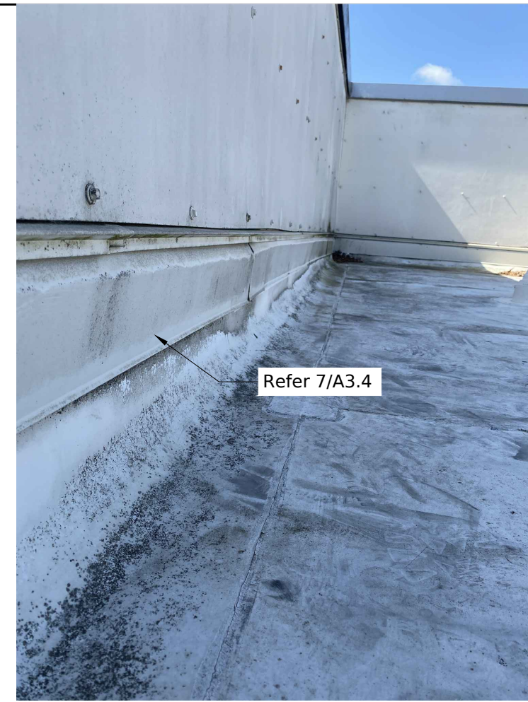
2 Piece Metal Counterflashing typ.
