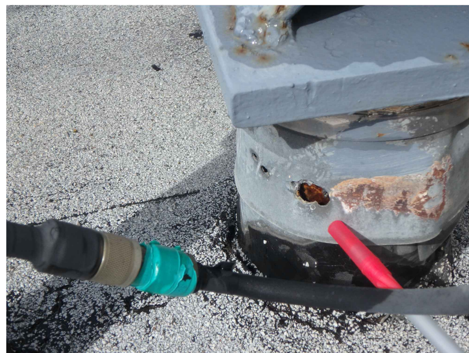
21 Typ. parapet support flashing Refer 3/A2.3
