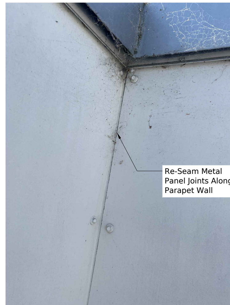
13 Metal panels at parapet wall corner
