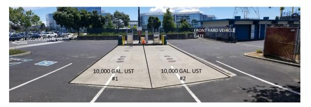
2. Two-5,000-gallon storage tanks in a covered, concrete vault immediately adjacent to and west of the lagoon pump station building (pump station) at the Corporation Yard. The tanks provide diesel fuel for vehicles and equipment via a single fuel dispenser and for the day tank inside the pump station.
