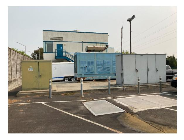
5. One-1,000-gallon underground storage tank (UGST) for diesel fuel located in the Bank of America (B of A) parking lot on the northeast corner of the intersection of Edgewater Boulevard and E. Hillsdale Boulevard. A 25-gallon day tank and an emergency generator are inside the B of A building. The emergency generator powers the traffic signal at the intersection and pumps in lift station 29. (As built plans available.)
