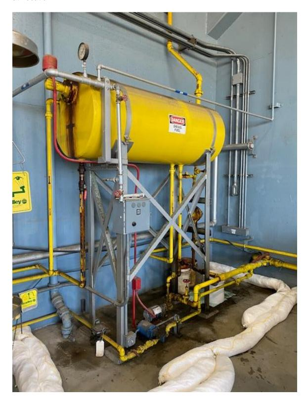
4. One-275-gallon day tank and 400-gallon subbase tank below the existing generator in an enclosure. The emergency generator powers the Corporation Yard including lift station 59.
