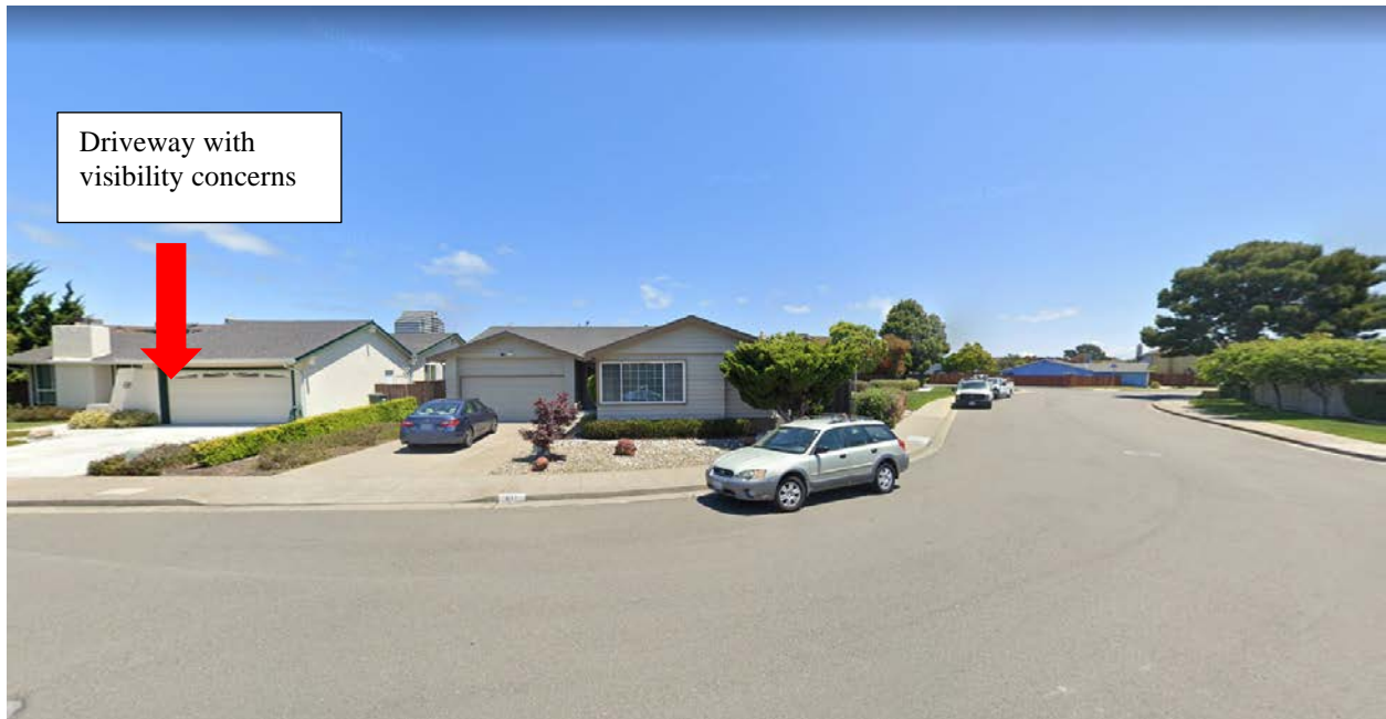
Existing condition at 611 Leo Drive looking east along Leo Drive
