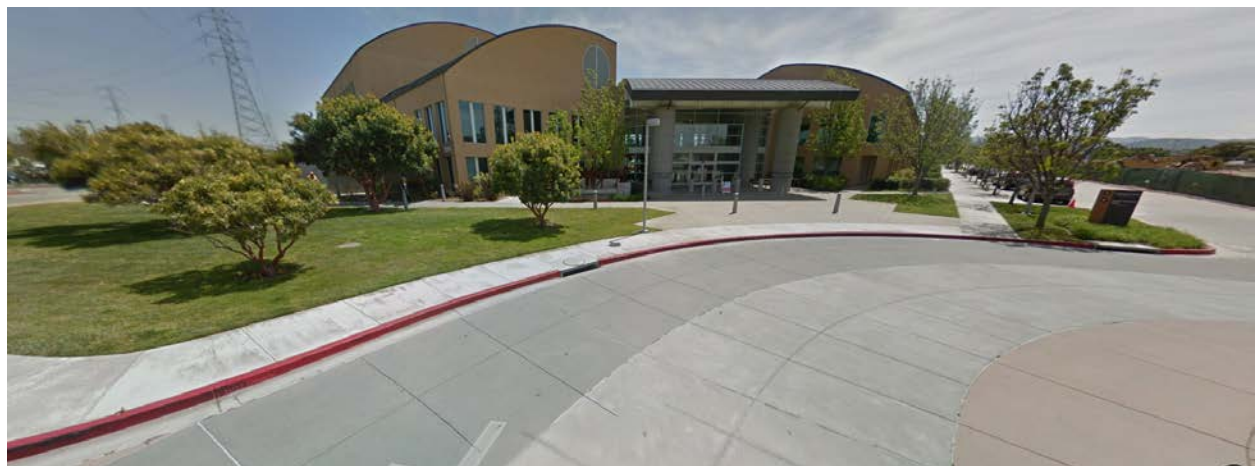
Existing Condition looking southbound
