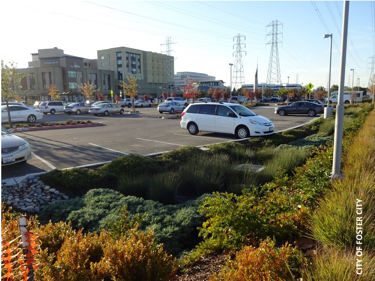
Bioretention area located along Foster City Boulevard.
