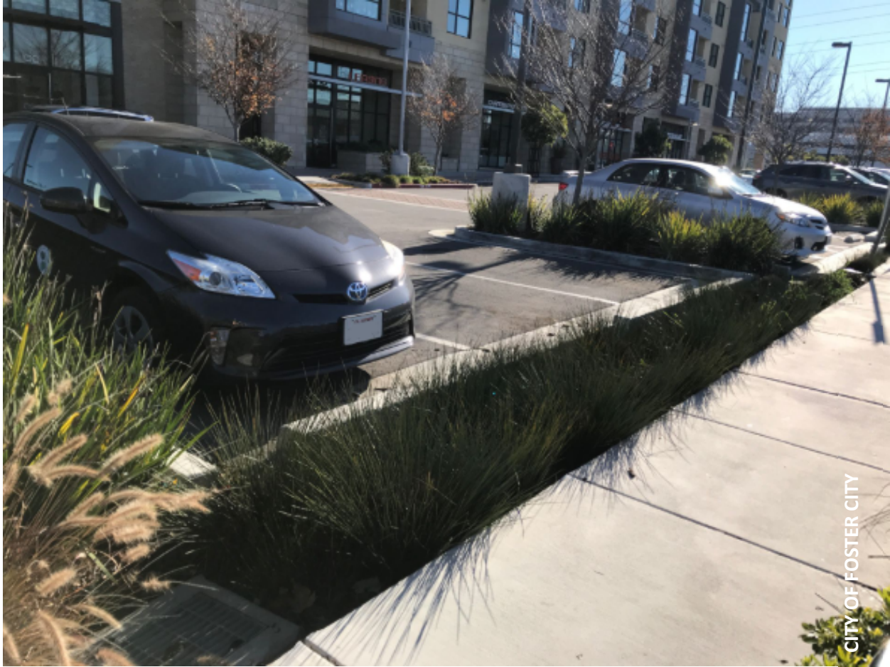
Bioretention area located at One Hundred Grand mixed-use commercial/residential development.
