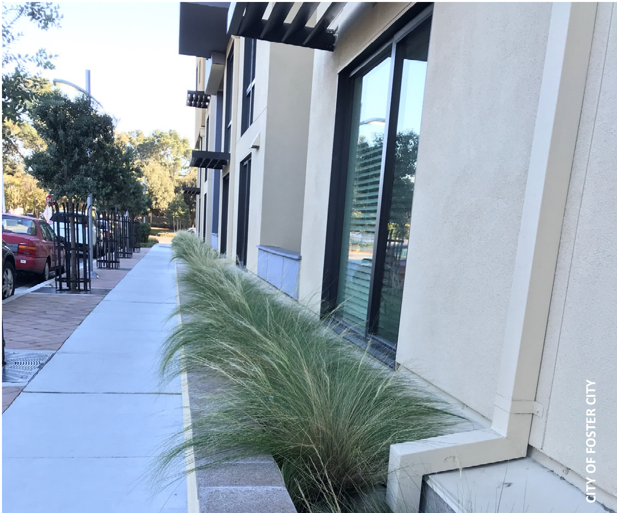
Flow-through planter at Triton Pointe.
