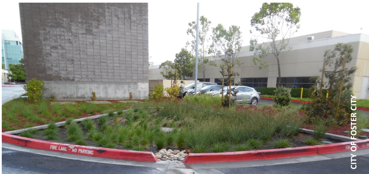
Bioretention area located at the Gilead Sciences Campus.
