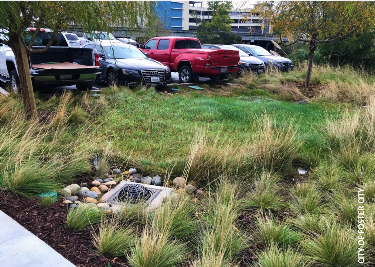
Bioretention area located at Lincoln Centre.
