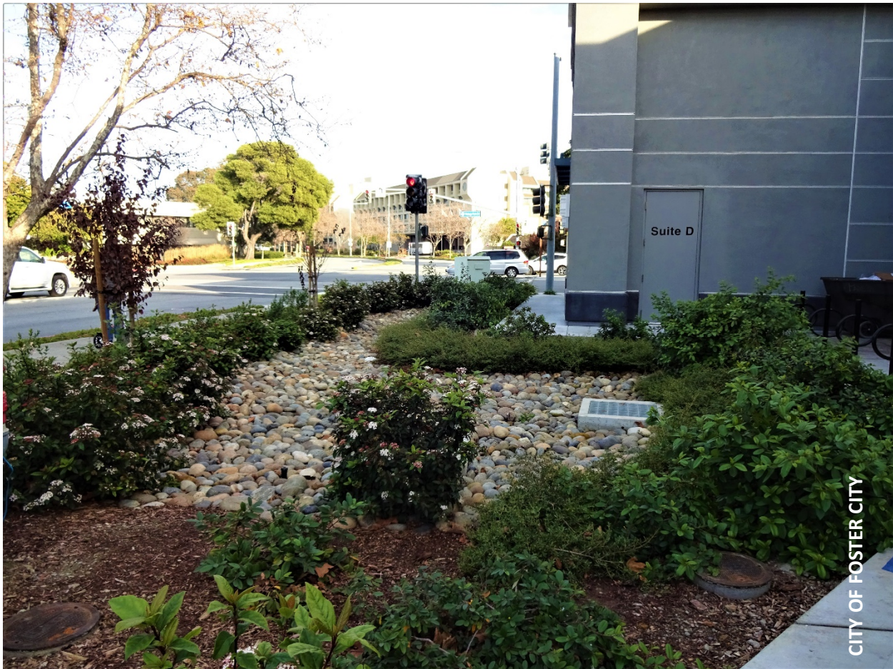
Bioretention area located at the TownePlace Suites, 1299 Chess Drive.
