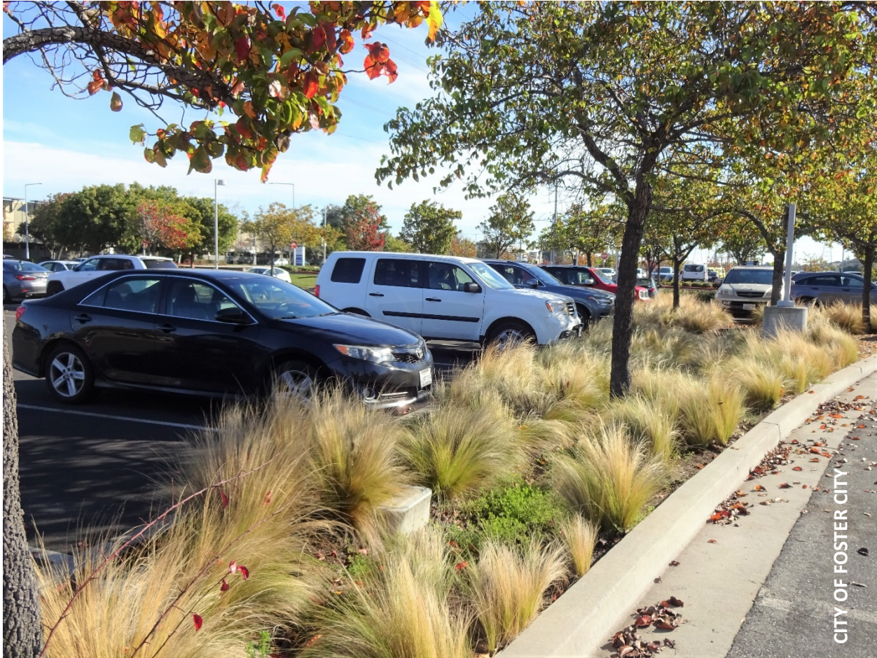
Bioretention area located at City Hall.
