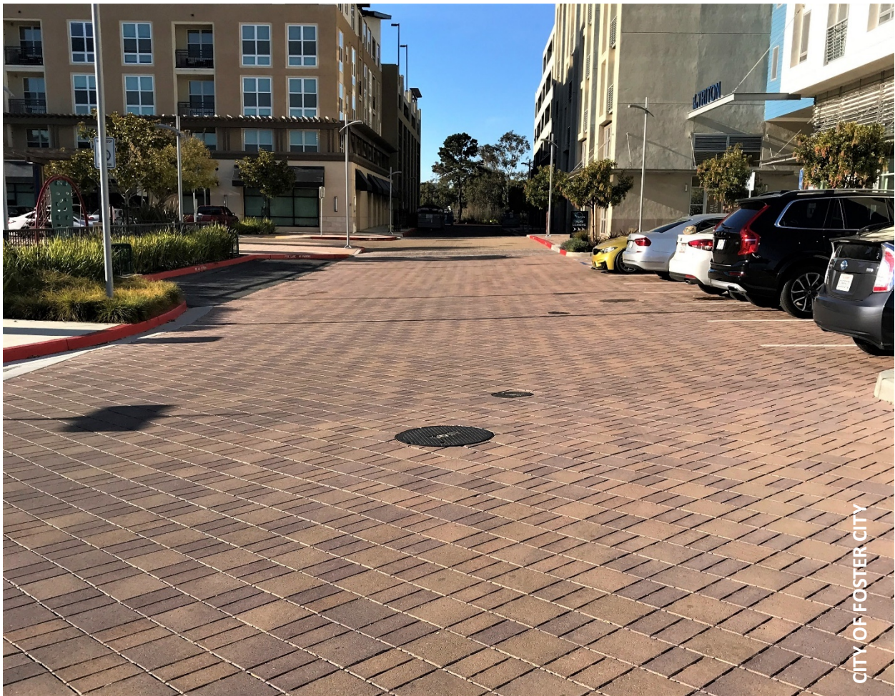
Permeable pavers located at The Triton Apartments.
