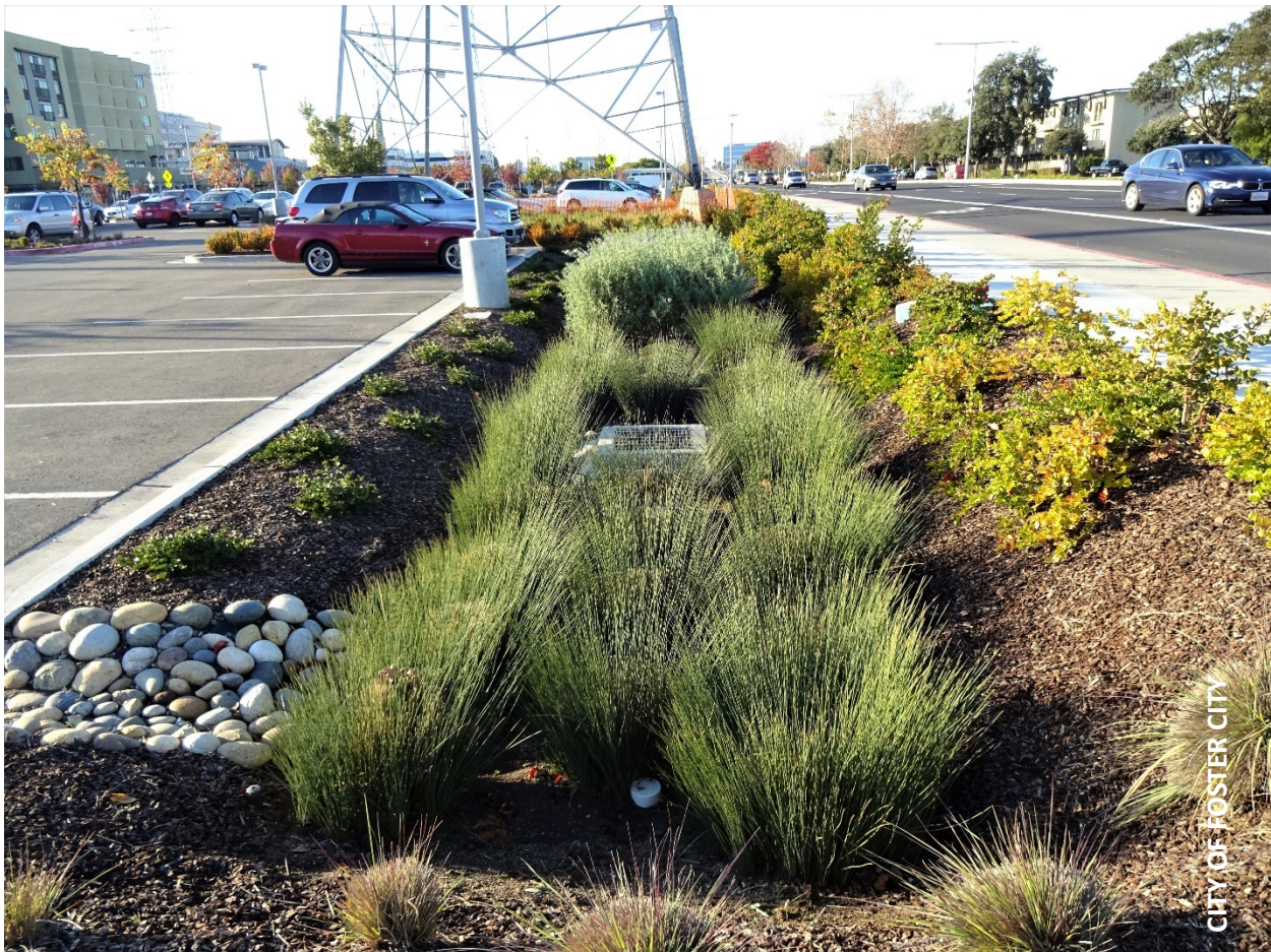
Bioretention Area at North Peninsula Jewish Campus.
