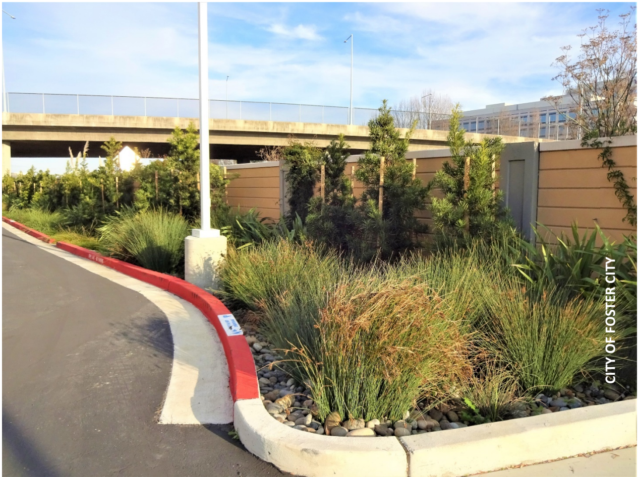
Bioretention area located at TownePlace Suites, 1299 Chess Drive.
