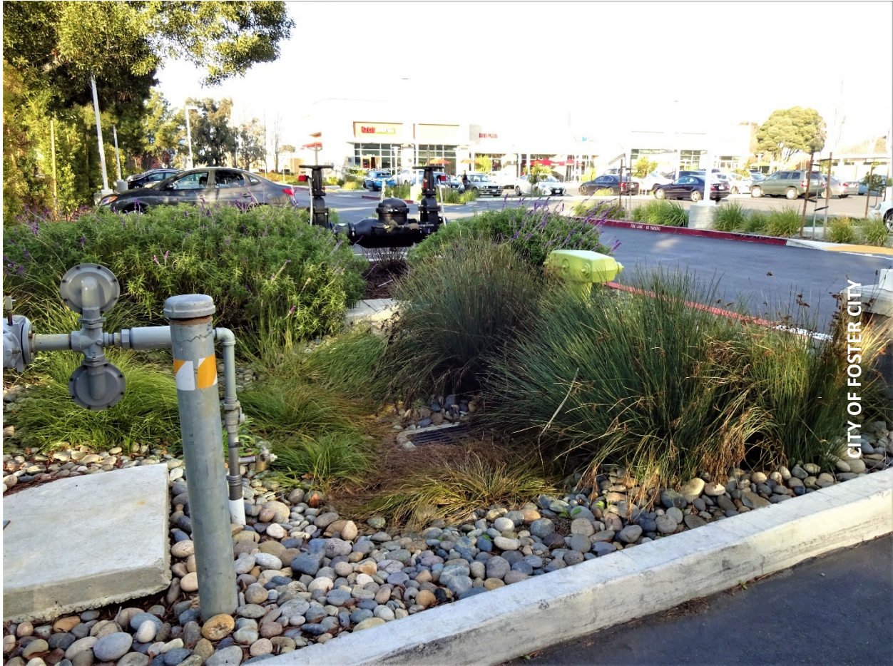
Bioretention area located at Foster City Hotel, Inc., Retail and Restaurant.
