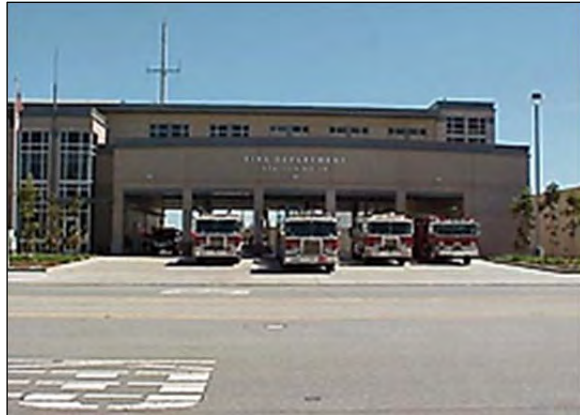
Foster City Fire Station
