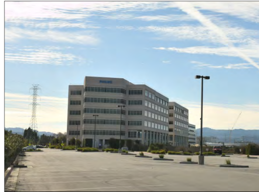
Bayside Towers and associated parking lot east of the project site
