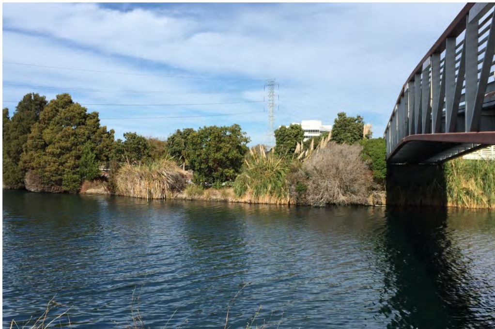
Views from the west toward the project site
