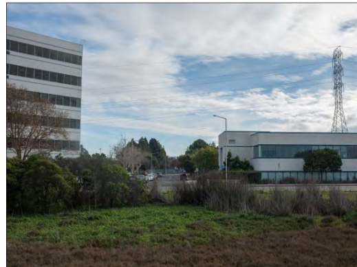
Lincoln Centre and Foster City Corporation Yard north of project site
