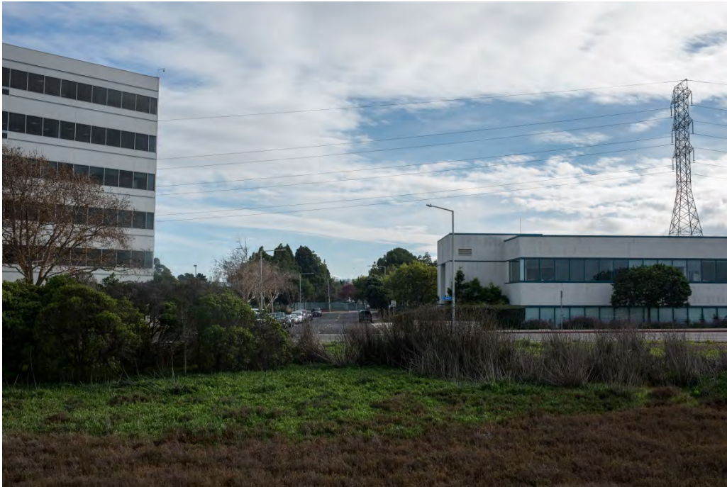
Views from the north towards the project site
