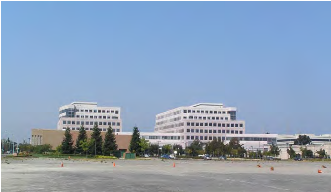
View from the Project Site towards the north, across Civic Center Drive.
