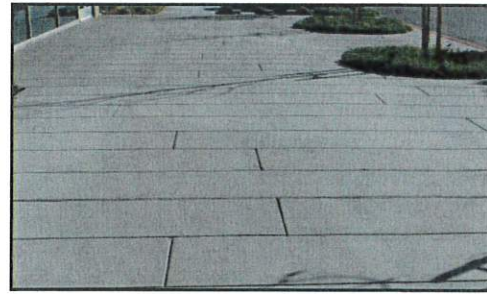
Fig 3.4a Example of paving materials
