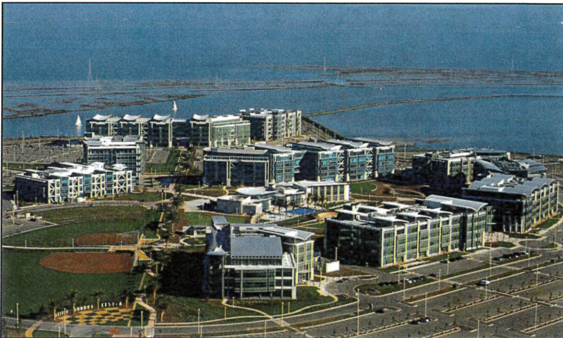
Fig 5.2 Example of building height hierarchies. Note the range in heights from the one story amenities building to the 5 story building office/R&D buildings.
