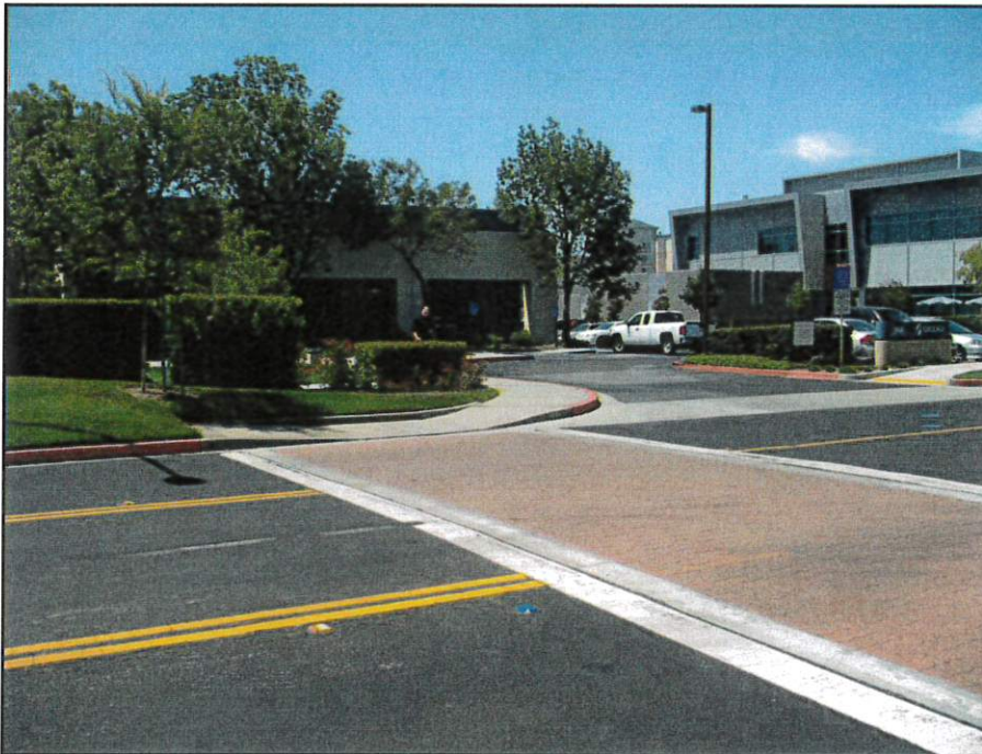
Fig 3.4c Example of clear demarcation – different paving materials –where walkway intersect with roadway
