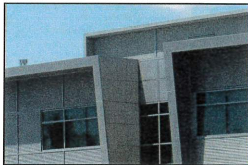
Fig 5.5b Metal panels and glazing
