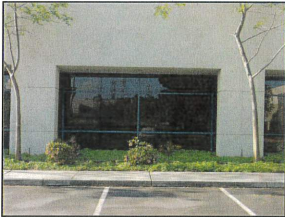
Fig 5.3g Arcade openings at ground floor
