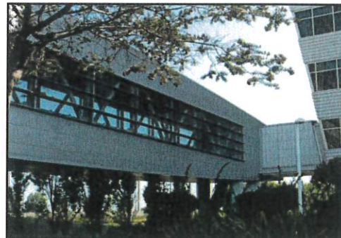
Fig 5.6c Example of skywalk at EFI campus
