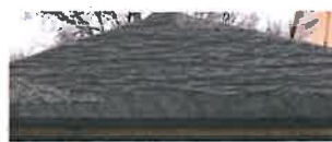
Conventional organic felts can absorb moisture, causing severe buckling and wrinkling—and a terrible-looking roof!
