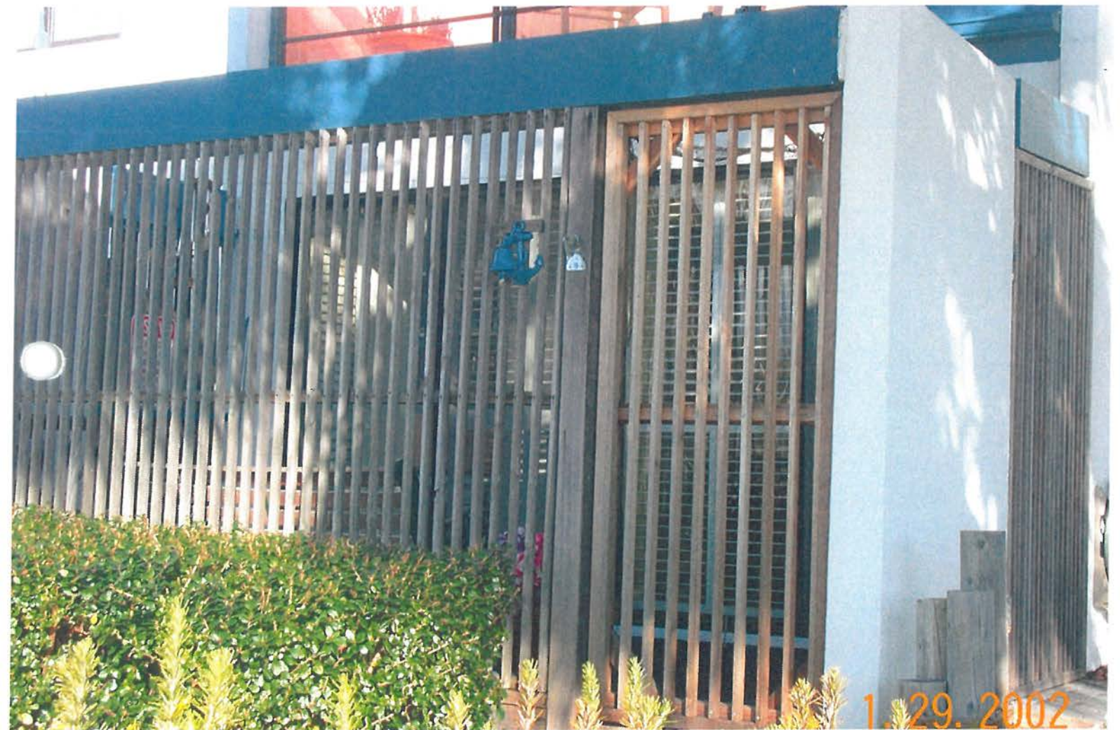
First Floor Enclosure at 926=OK
