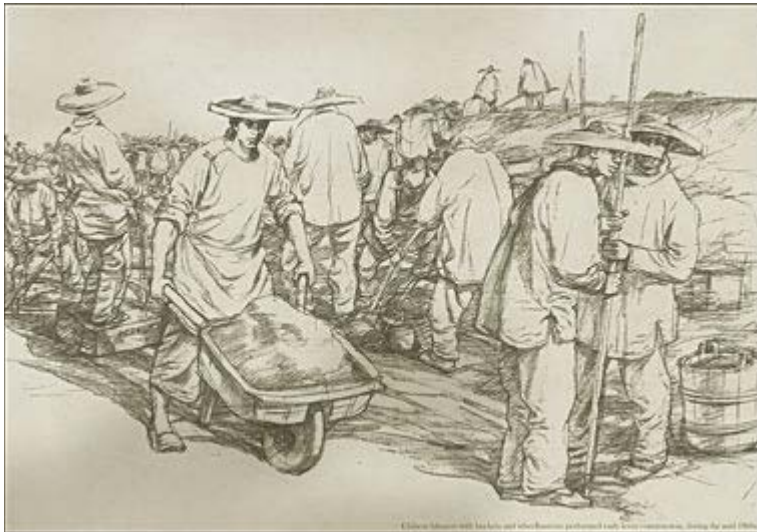
Figure 2. An illustration of Chinese laborers constructing levees in the San Francisco Estuary. From Family Water Alliance 2012.
