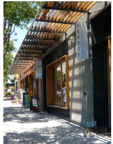
3.1a Unique storefronts and custom sunshades or awnings strongly encouraged; integrate blade signs
