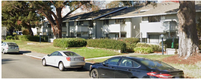
Beach Cove Apartments
