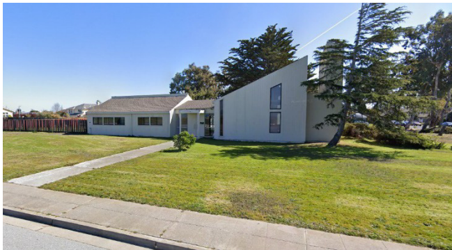
1601 Beach Park Boulevard Existing Building
