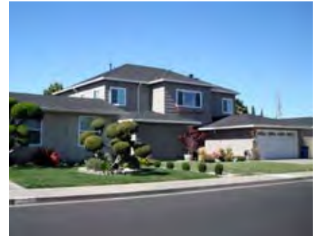
Examples of homes with second-story additions in Foster City.
