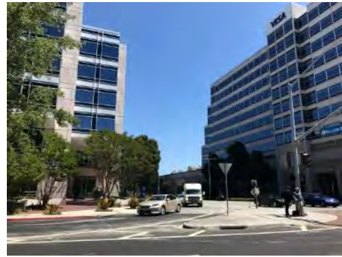
Photo 4– Midrise office buildings
