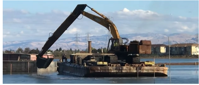
Lagoon dredging to remove sediment mitigate flood risk.
