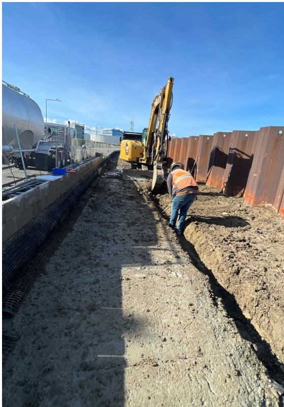
Levee retaining wall under construction
