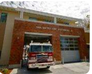
San Mateo Station 24— 319 S. Humboldt St. Engine 24—3 personnel
