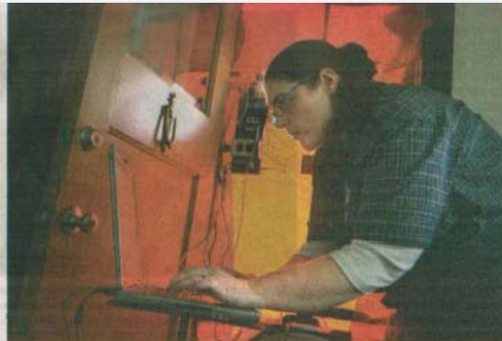
Chris Maki from Green Build Technology uses a blower door to depressurize a home and test the estimated cost of air leakage during a home energy audit. Ben Woloszyn/Boomerang photographer
