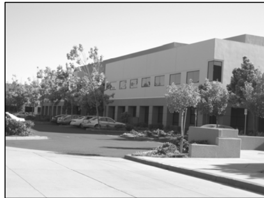
Photo V.A-1: Typical project site office building
