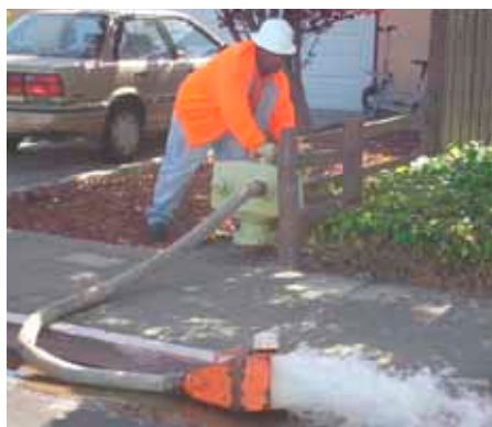
Fire Hydrant Flushing
